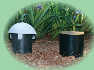
Your sewer relief valve (SRV) protects your home from costly sewage backups. Check your SRV after storms to ensure that branches and debris are not preventing proper operation. For peace of mind, call us at 373-1274 for a free inspection.
